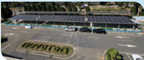
▲ Expansion of solar panels in the parking lot of the Yanshin Plant
